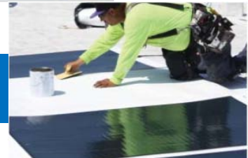
Peel & Stick Modules to TPO
