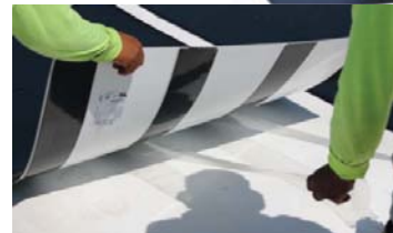
Peel & Stick Modules to TPO
