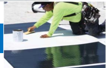
Peel & Stick Modules to TPO
